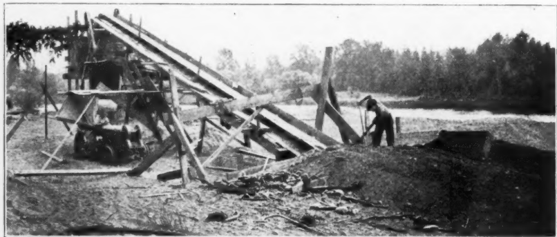
Scraper Discharge and Incline to Plant
